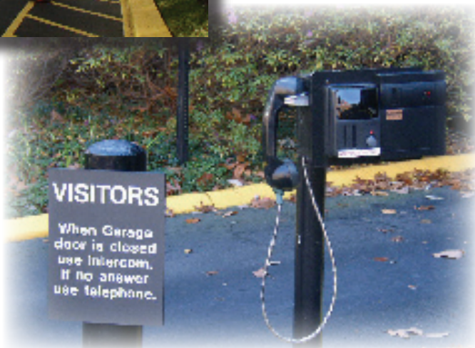
A video entry system provides security for a remote parking deck.
